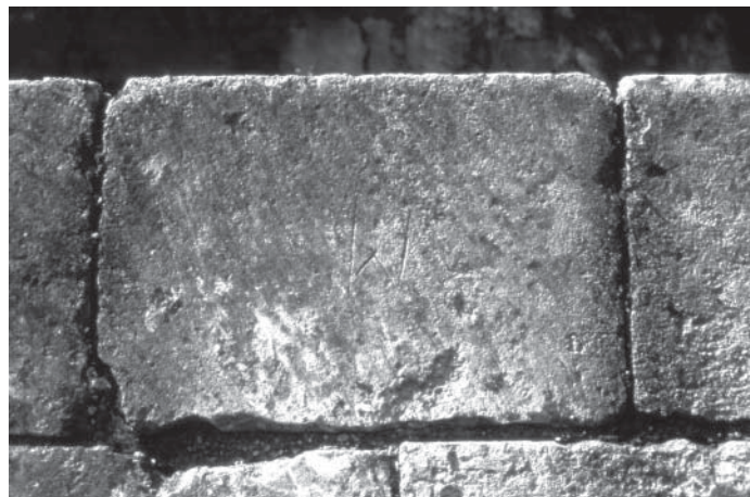
FIG. 5 Roche Abbey, mason's mark on nave N. aisle wall. Photograph: J. S. Alexander.
